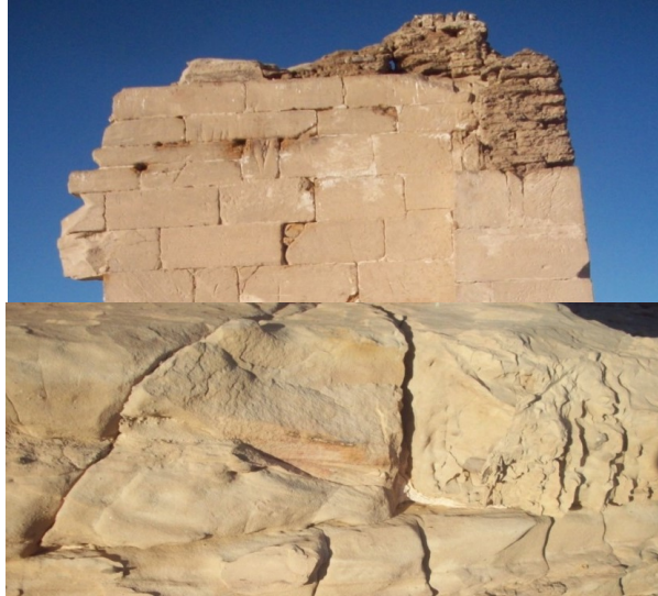
Fig. 4. A, B. Longitudinal single cracks on the wall of El-Nadira Temple, millimeters in width and centimeter in length, due to arid climate and wide range of temperatures.
