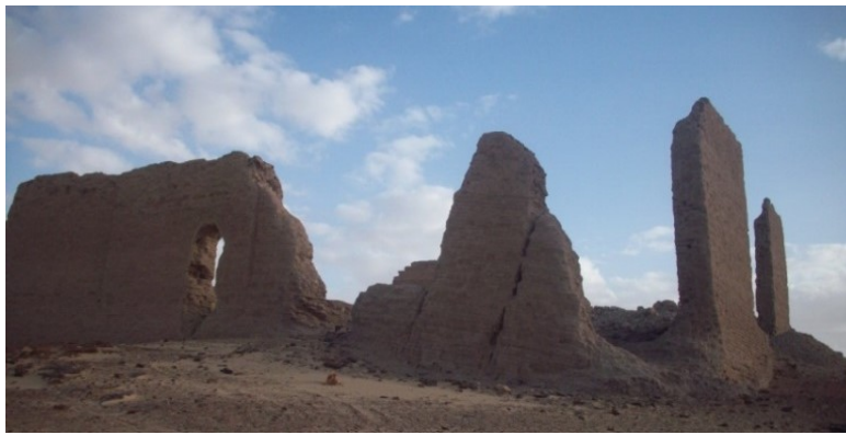
Fig. 9. The presence of structurally unstable walls at El-Nadira Temple as a result of physical weathering (natural causes), or constructional causes
