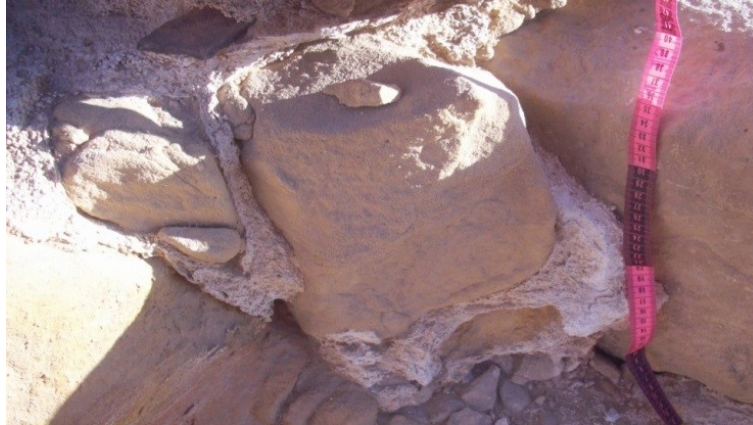
Fig. 13. Disintegration of the mortar used in jointing the stones wall at El-Nadora Temple as result of climate conditions
