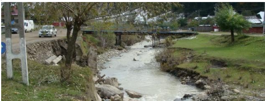
Figure 3. Upstream view of the Tazlaul Sarat riverbed in research area P1, year 2016 (Luca, 2016).
