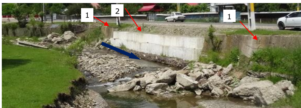
Figure 5. General view of the rehabilitation of the bank defence at research point P1: 1 – initial plain concrete retaining wall; 2 – sector rehabilitated with a gabion retaining wall (author's photo, 2019).
