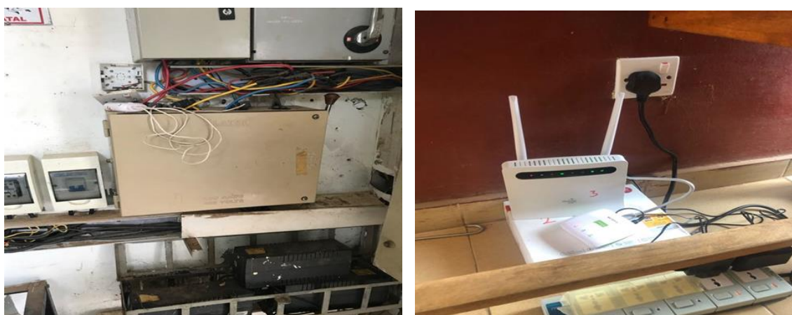
Figure 2. Pictorial view of the efergy Transmitter connected to the transfer switch and the efergy router connected to a meter in the admin block.
