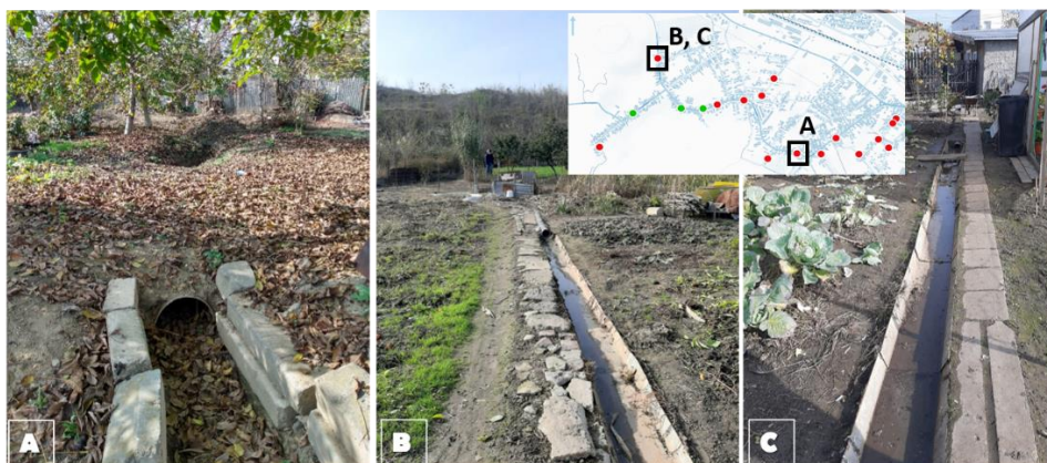
Figure 9: Pipes unearthed from the old sewerage system on Calea Giulești (6 Nov 2020)
